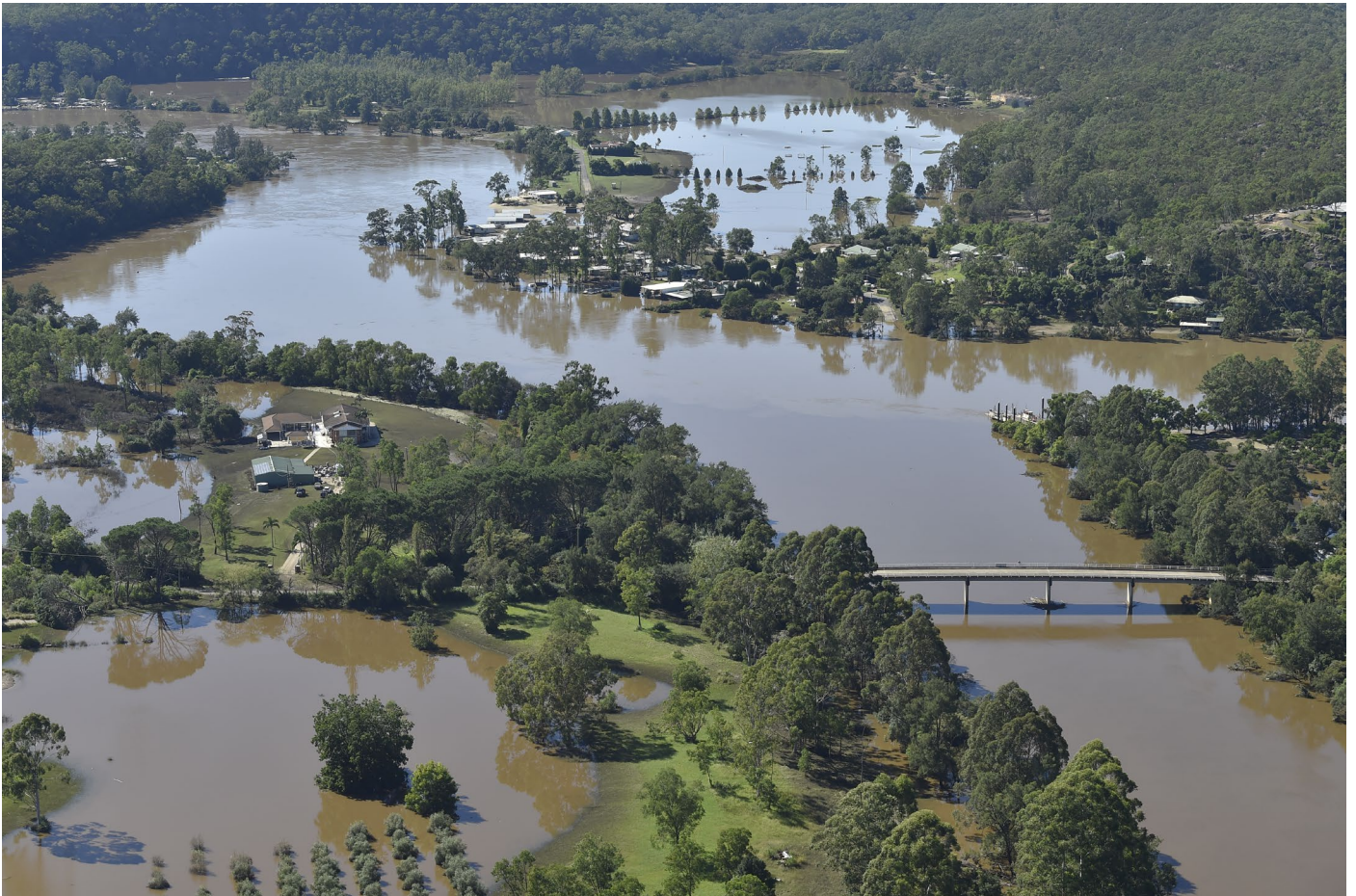
Junction of Colo and Hawkesbury Rivers, 2021 flood. Photo by Adam Hollingworth, courtesy of INSW
