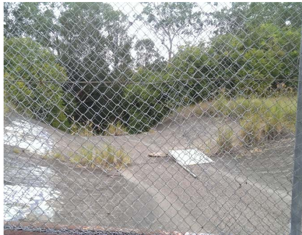
Photograph 5: Concrete drainage structure leading to creek
