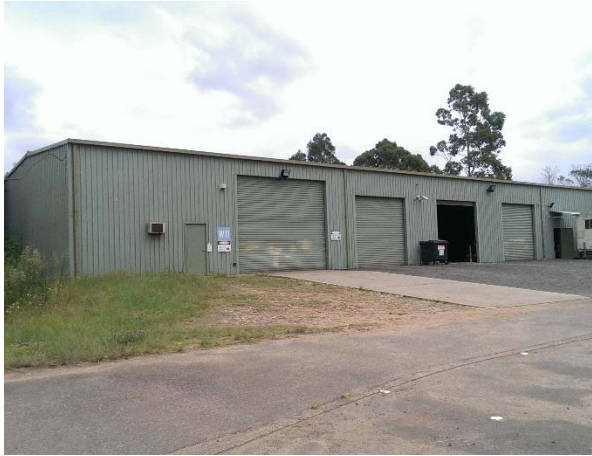
Photograph 19: W11 Colourbond steel warehouse
