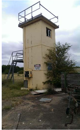
Photograph 8: W02 Radar room (2 storey building with deck on top)
