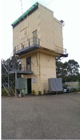
Photograph 7: W02 Radar room (3 storey building)
