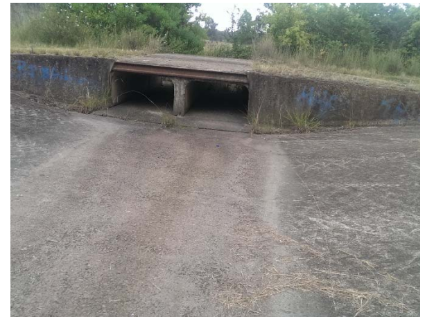
Photograph 6: Concrete culvert on drainage structure
