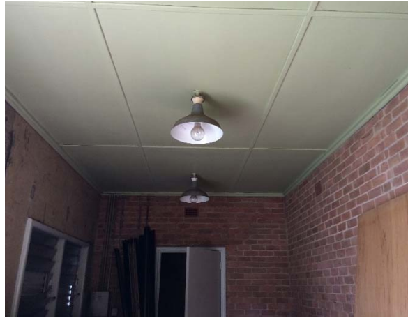
Photograph 50: Interior of Building X7
