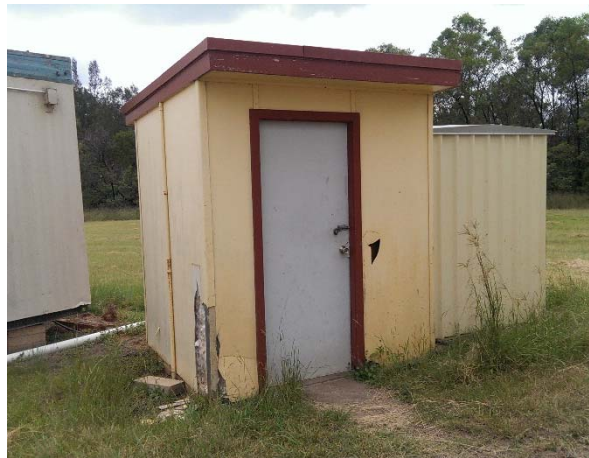
Photograph 17: Toilet adjacent to W10
