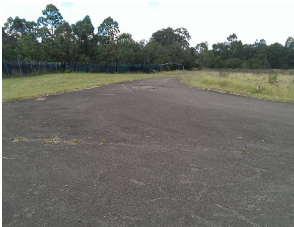
Photograph 34: Intersection 1 on Stage 4 facing southwest (bitumen paved road)
