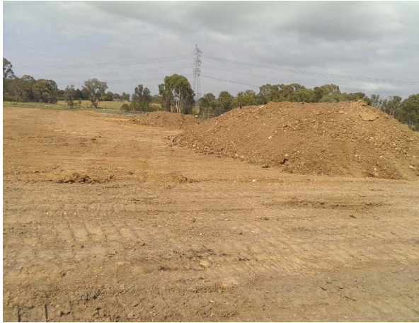
Photograph 1: Stockpile area on Building X1 footprint facing southwest
