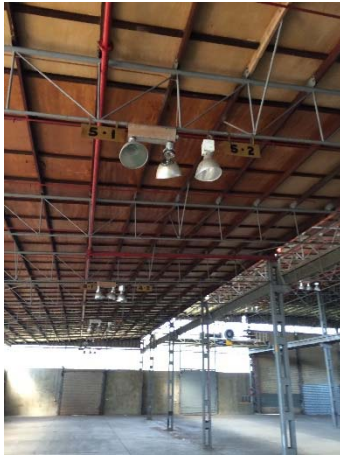
Photograph 49: Interior of Warehouse X2
