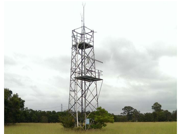
Photograph 12: W01 (south) steel frame structure
