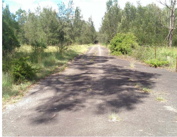
Photograph 38: Intersection 2 on Stage 4 facing southwest (bitumen paved road)
