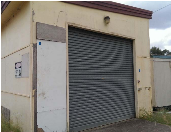
Photograph 16: W10 Empty garage space
