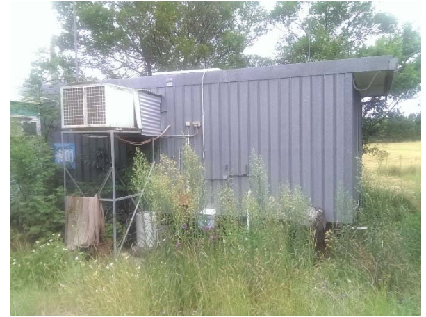
Photograph 27: W01 Portable storage shed
