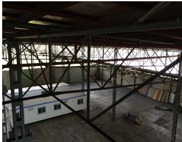
Photograph 53: Interior of Warehouse X1
