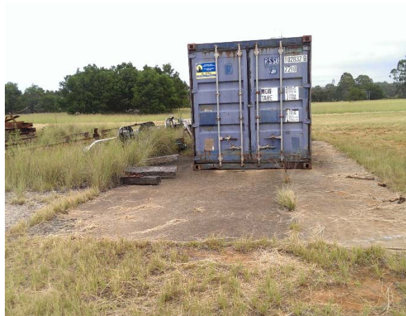
Photograph 11: Concrete slab (footprint of former W09 structure)
