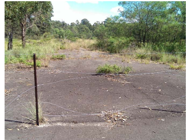
Photograph 36: Intersection 2 on Stage 4 facing southwest (bitumen paved road)
