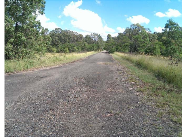
Photograph 33: Bitumen paved road on Stage 3 facing northeast
