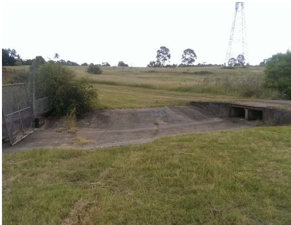
Photograph 4: Concrete drainage structure to the southwest of Building X1 footprint
