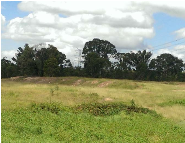
Photograph 46: Stockpile 31 containing road base overgrown with grass
