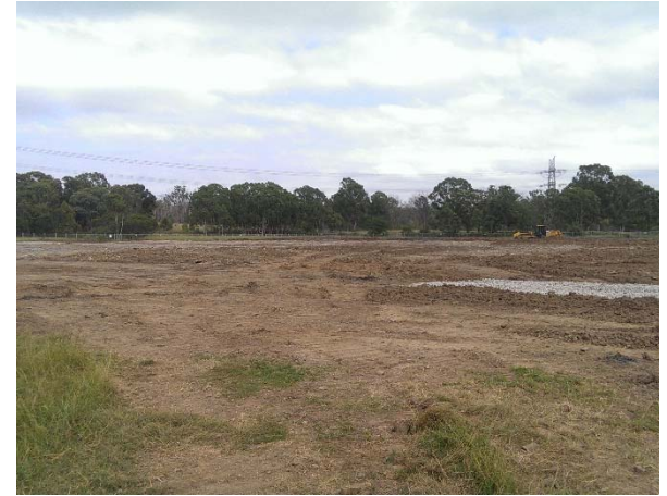
Photograph 3: Building X2 footprint facing west
