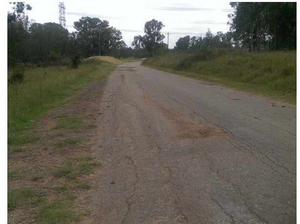
Photograph 30: Stage 1 Road facing southeast
