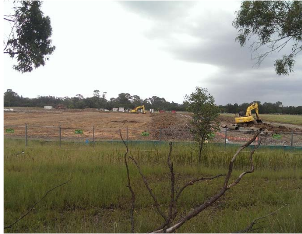
Photograph 2: Stockpile area on Building X2 footprint facing northeast
