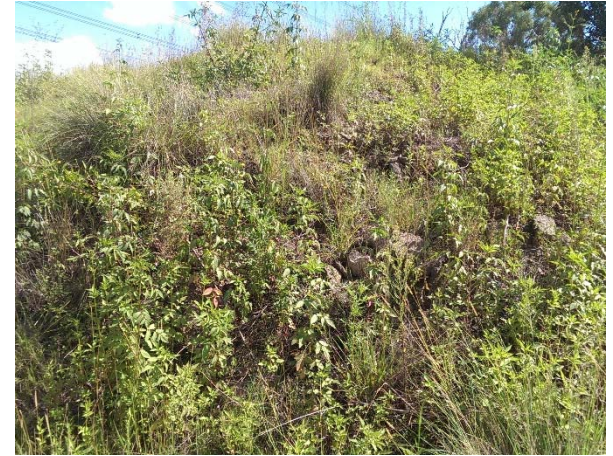
Photograph 45: Stockpile 32 containing road base overgrown with vegetation
