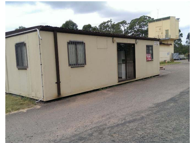
Photograph 24: Portable building opposite W11
