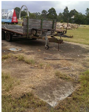
Photograph 10: Concrete slab (footprint of former W09 structure)
